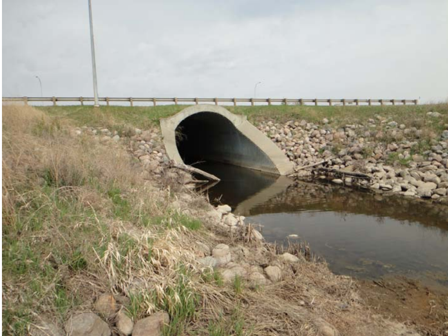
Photo 7 – CSP culvert beneath eastbound lanes of Highway 15 at Astotin Creek – BF73649
