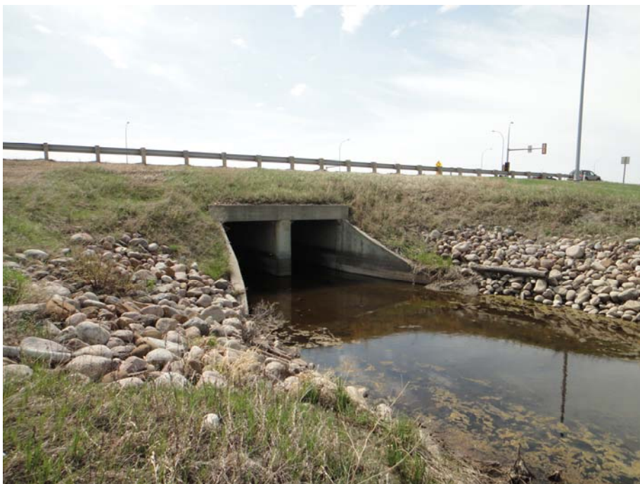
Photo 8 – Double box culvert beneath westbound lanes of Highway 15 at Astotin Creek - BF73649
