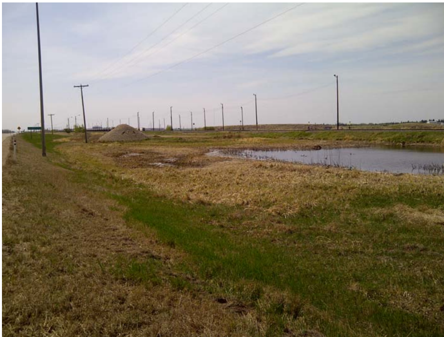
Photo 6 – Standing water and poor drainage between north embankment of Highway 15 and parallel CNR railway, looking west from the intersection with Range Road 220
