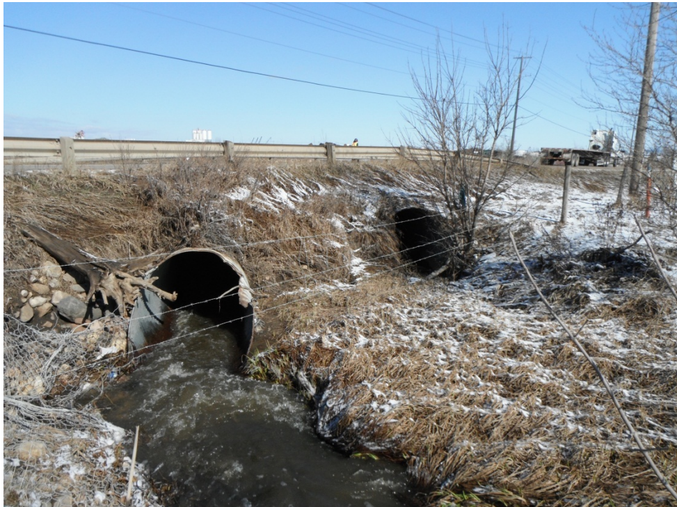
Photograph 13: Goldbar Creek, proposed crossing site, downstream view to culvert inlet on the east side of 34 Street (note overflow culvert).
