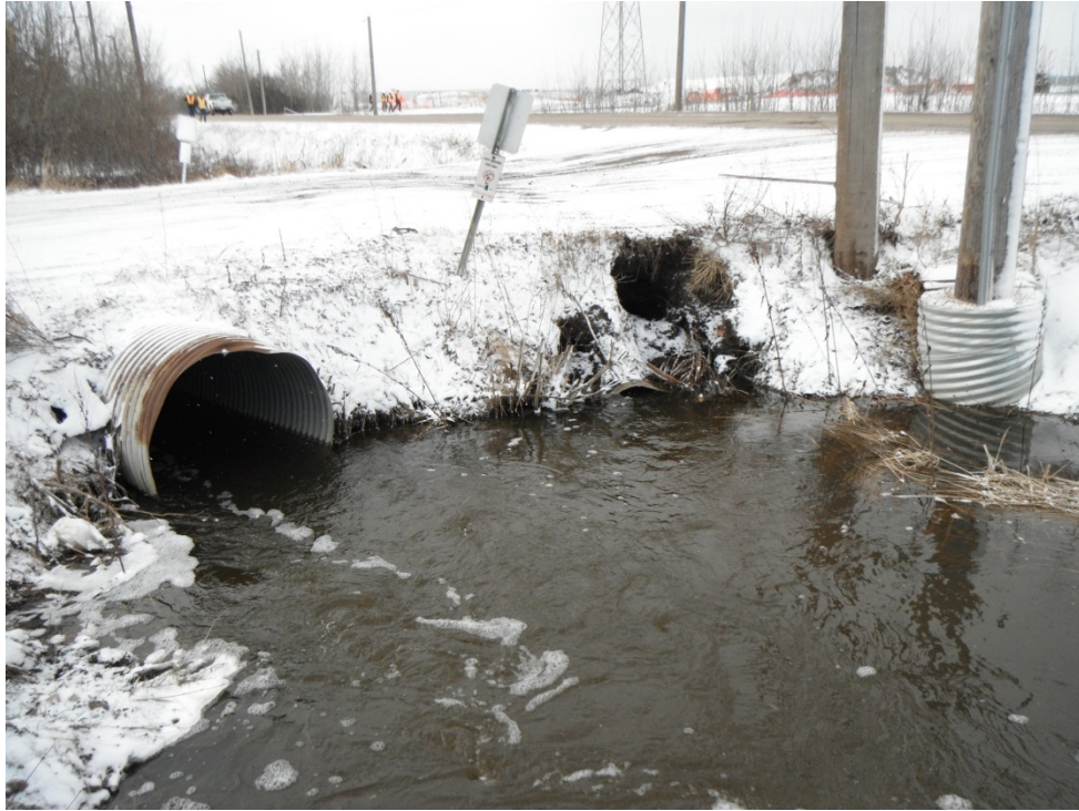
Photograph 5: Fulton Creek, driveway access culvert outlets, upstream view.
